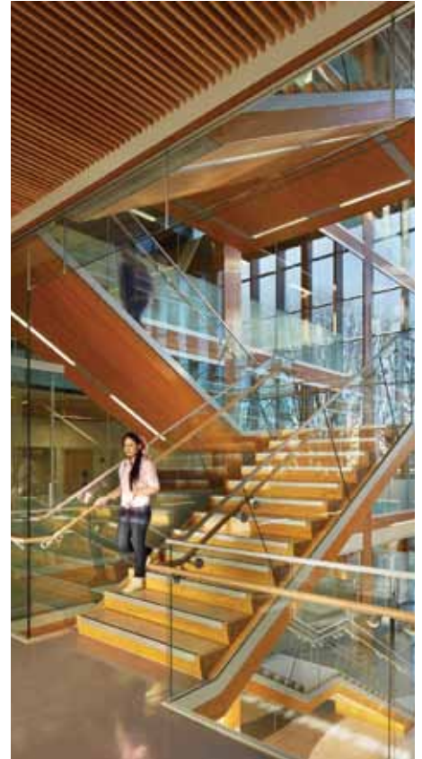
Cantilevered atrium stair at UBC Earth Sciences Building. Courtesy of Martin Tessler.
