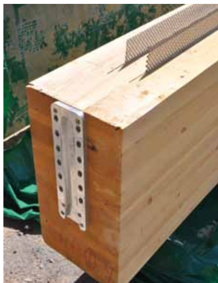
Pre-engineered dovetail connection and HSK wood concrete composite connection at the UBC Earth Sciences Building. Courtesy of Equilibrium Consulting.
