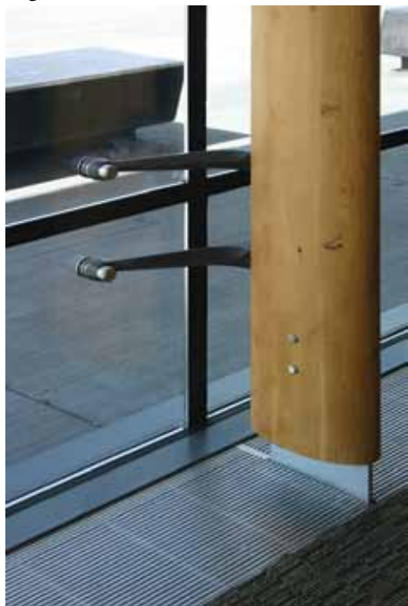
Stainless tight-fit dowels and steel castings at the Prince-George Airport. Courtesy of MacFarlane Green Architecture.
