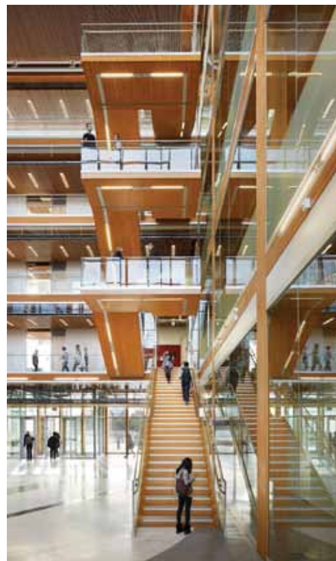
Cantilevered atrium stair at UBC Earth Sciences Building. Courtesy of Martin Tessler.
