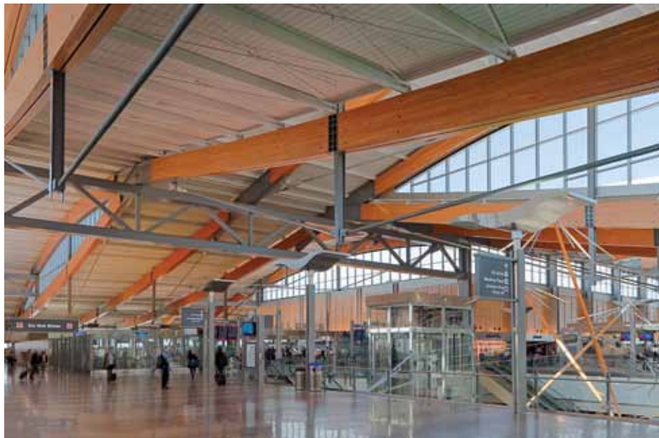
Terminal 2 at the Raleigh Durham Airport with BVD moment connections. Courtesy of Brady Lambert.
